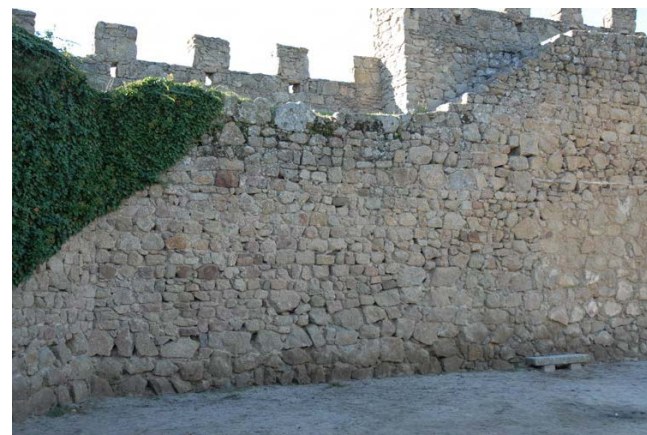
Tramo 24, intramuros, arranque
