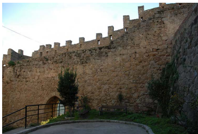
Tramo 22, intramuros, general
