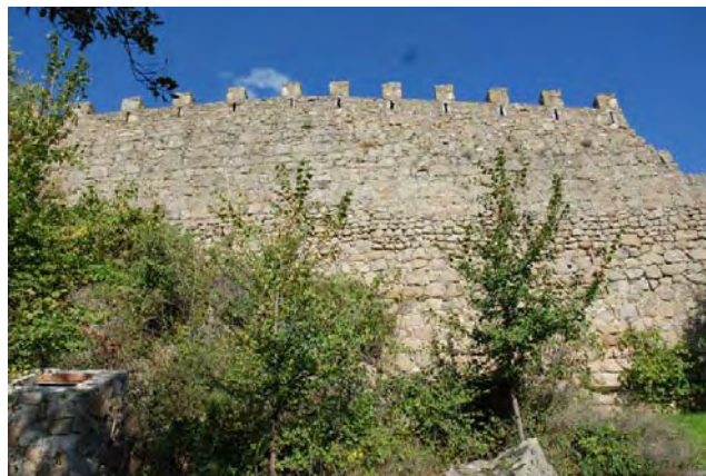
Tramo 18, extramuros, arranque
