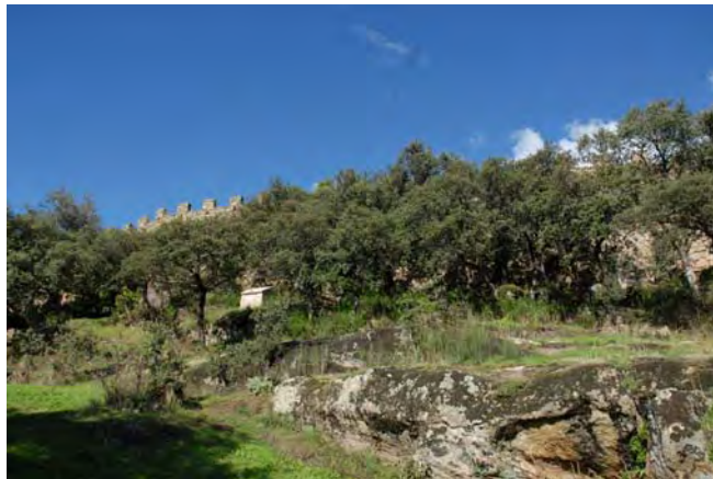
Tramo 16, extramuros, zona final
