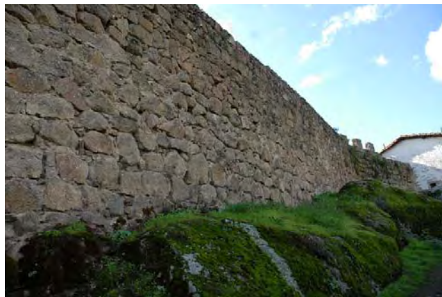
Tramo 16, intramuros, zona intermedia
