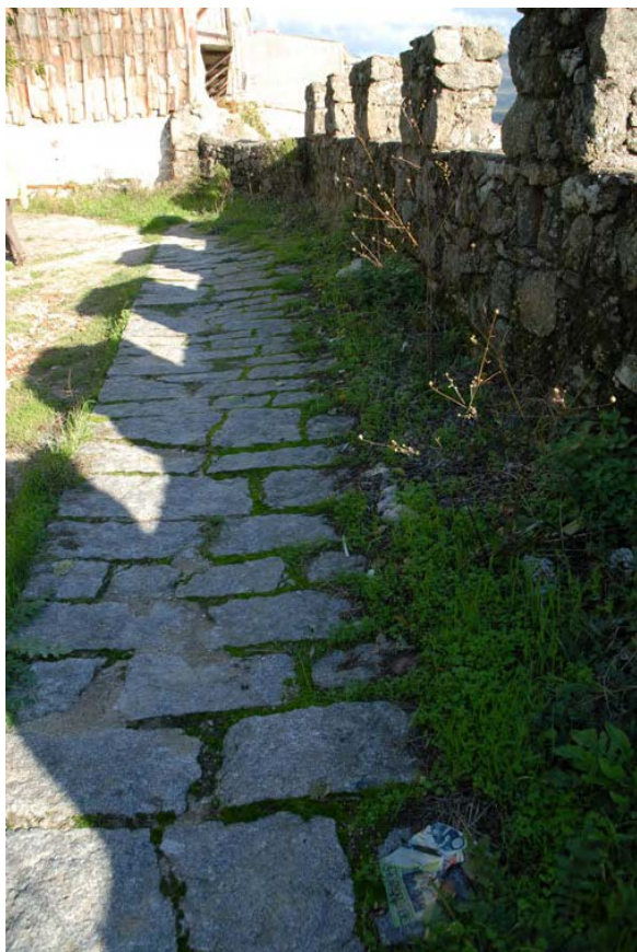
Tramo 12, intramuros, detalle adarve
