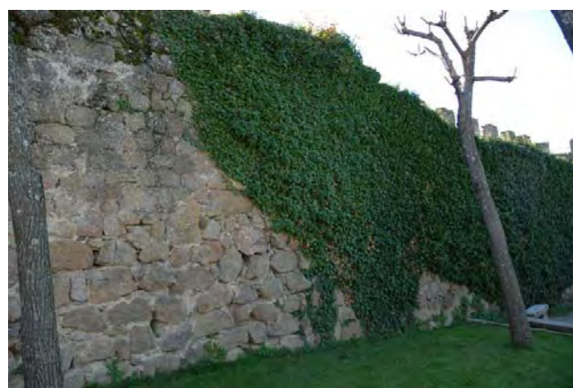
Tramo 23, intramuros, zona intermedia
