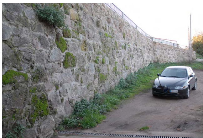
Tramo 31, extramuros, arranque
