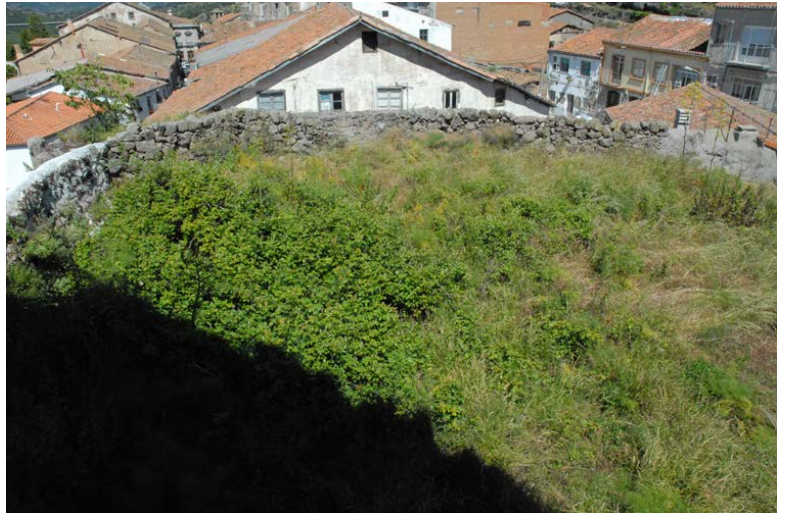
Tramo C1. Intramuros, adarve
