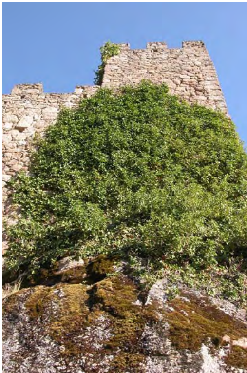
Tramo 25, extramuros, torre esquina
