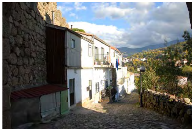
Tramo 14, extramuros vista general
