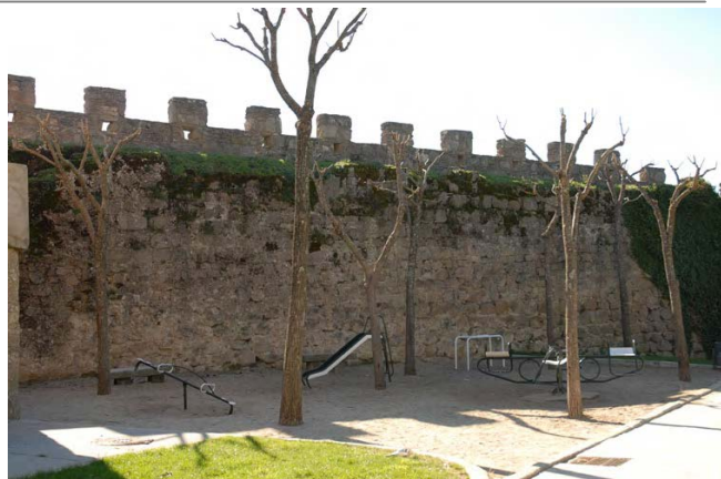
Tramo 23, intramuros, arranque
