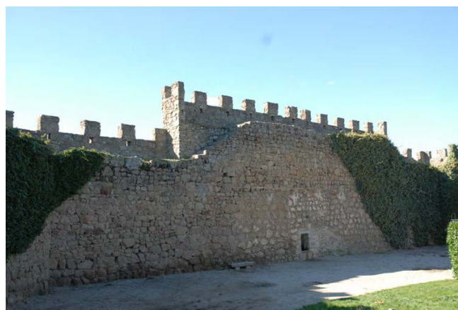
Tramo 24, intramuros, general
