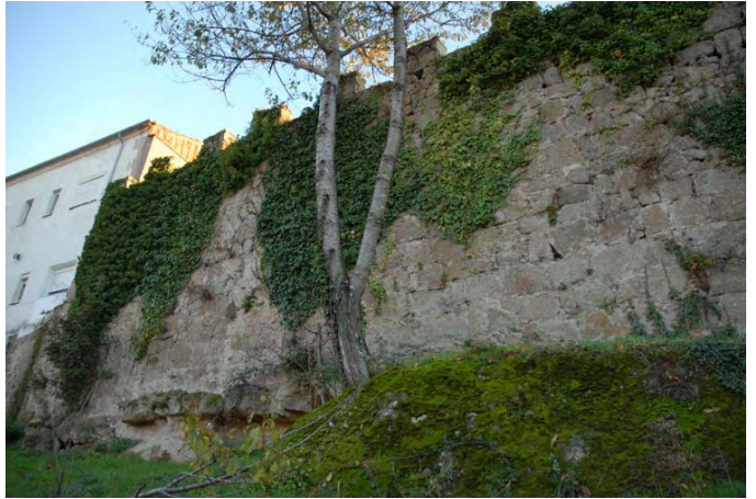
Tramo 26, extramuros, zona final
