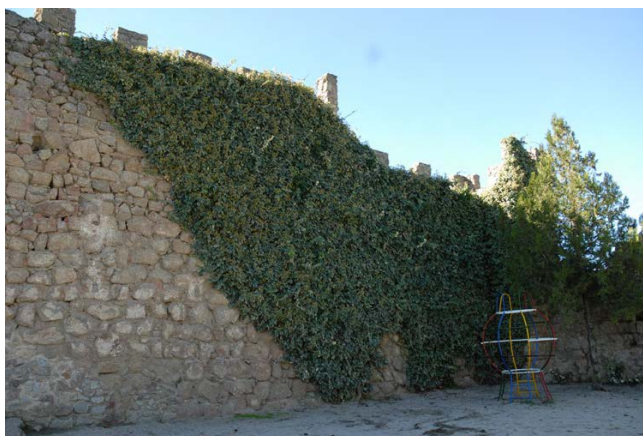
Tramo 24, intramuros, zona final
