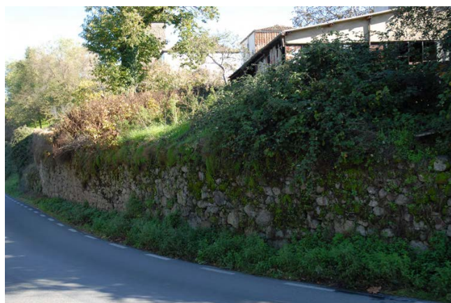
Tramo 28, extramuros, arranque
