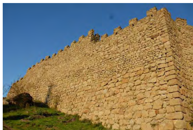
Tramo 24, extramuros, arranque
