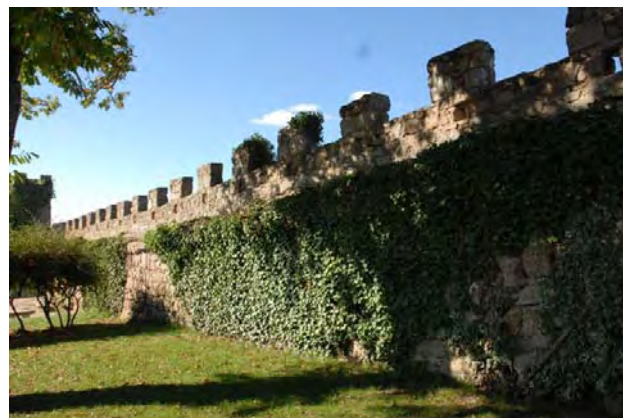
Tramo 25, intramuros, general
