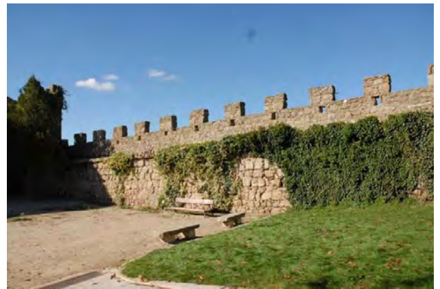
Tramo 25, intramuros, arranque
