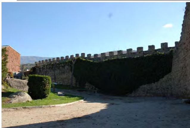
Tramo 23, intramuros, general
