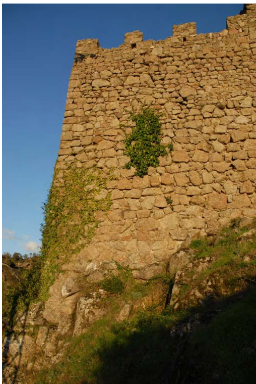
Tramo 24, extramuros, zona final
