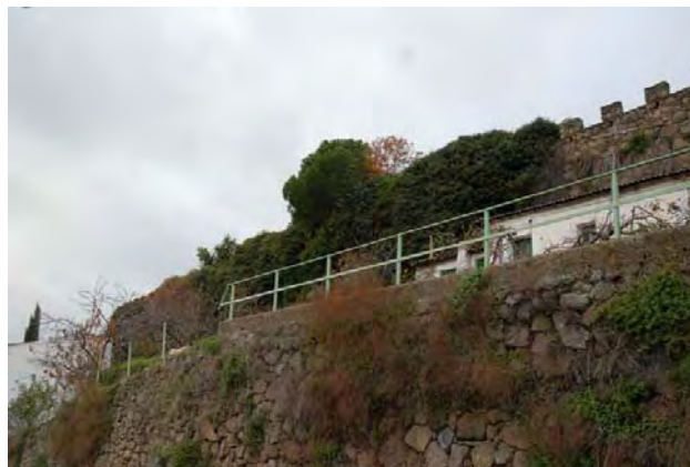
Tramo 12, extramuros, vista general
