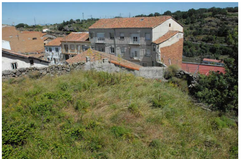
Tramo C1. Intramuros, adarve
