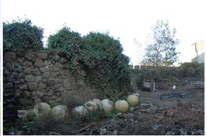
Tramo 40, intramuros, general
