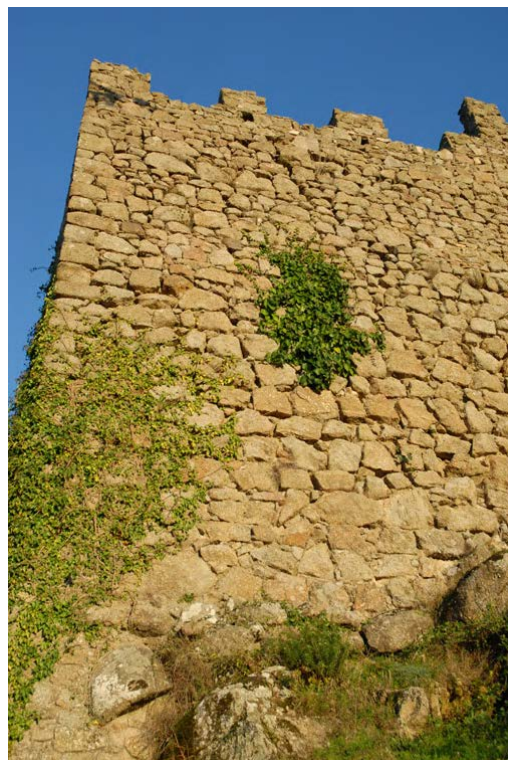
Tramo 24, extramuros, detalle torre esquina final
