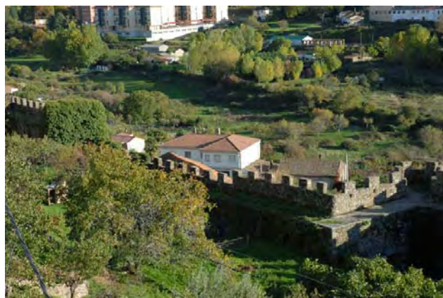
Tramo 14, intramuros, vista general
