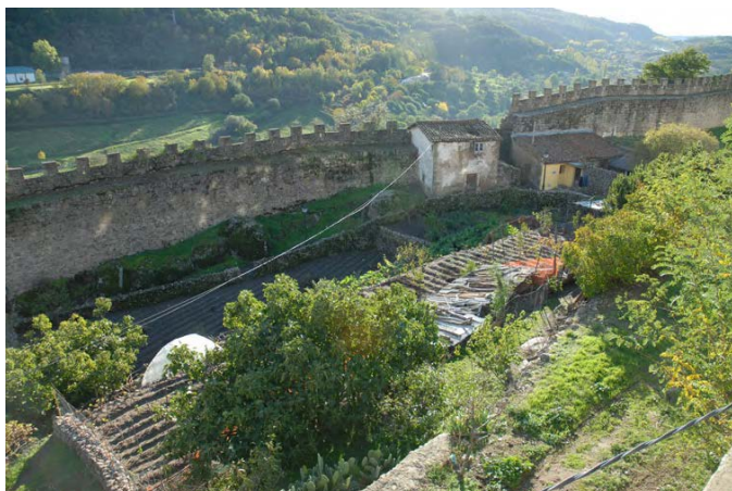
Tramo 16, intramuros, zona final
