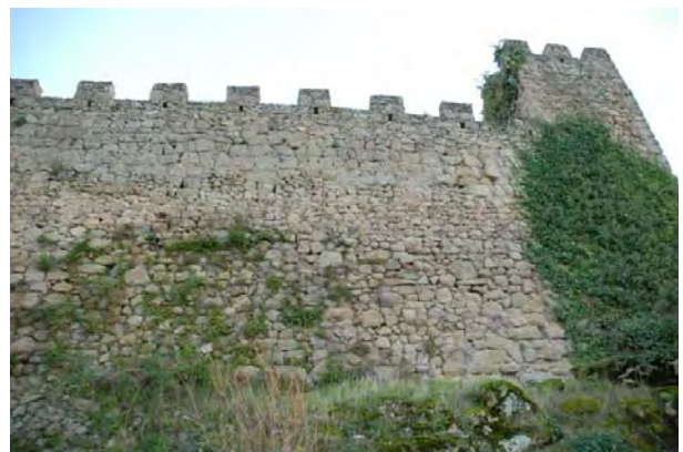
Tramo 25, extramuros, arranque
