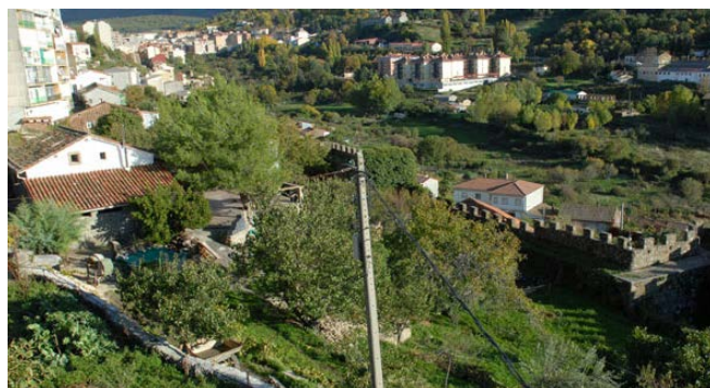
Tramo 13, intramuros, vista general
