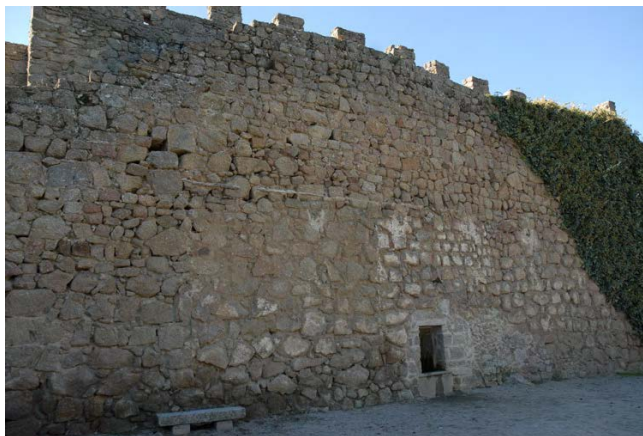
Tramo 24, intramuros, zona intermedia
