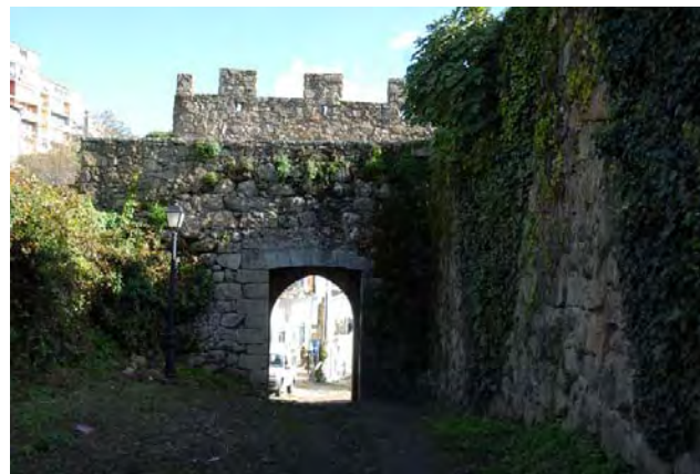
Tramo 15, intramuros, general
