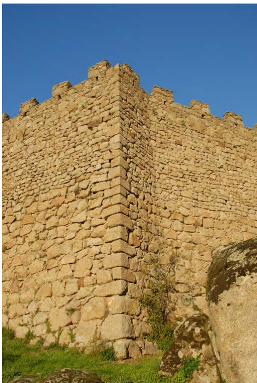
Tramo 23, extramuros, esquina
