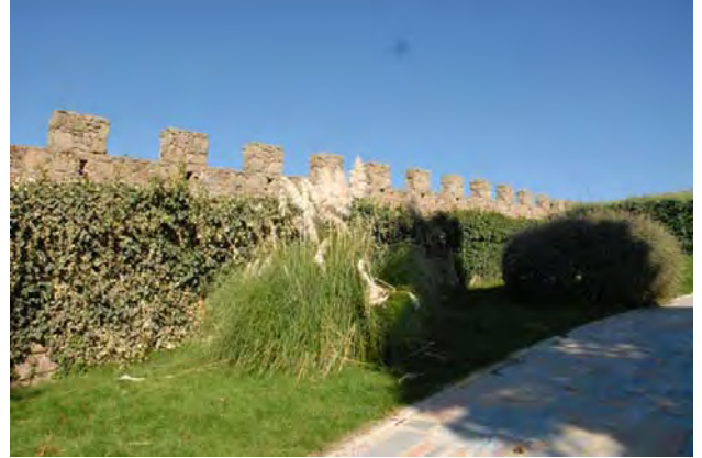
Tramo 25, intramuros, zona final
