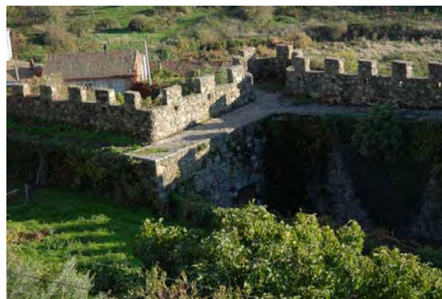
Tramo 15, intramuros, adarve
